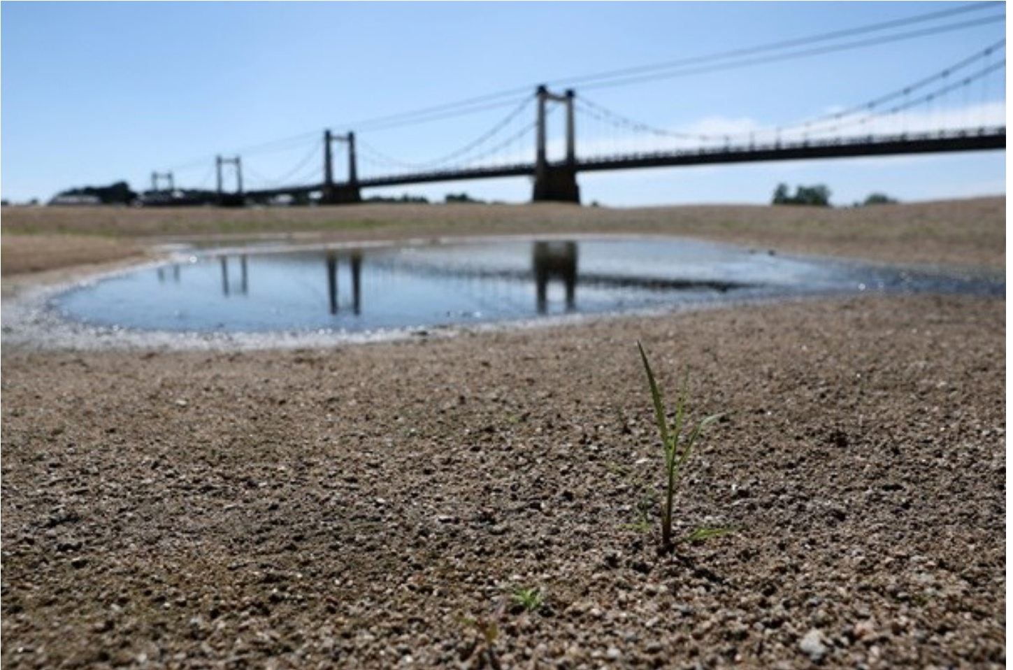
A plant in a branch of the Loire River in Montjean-sur-Loire as drought conditions worsen following a heatwave and water shortages across much of France, July 20. REUTERS/Stephane Mahe
